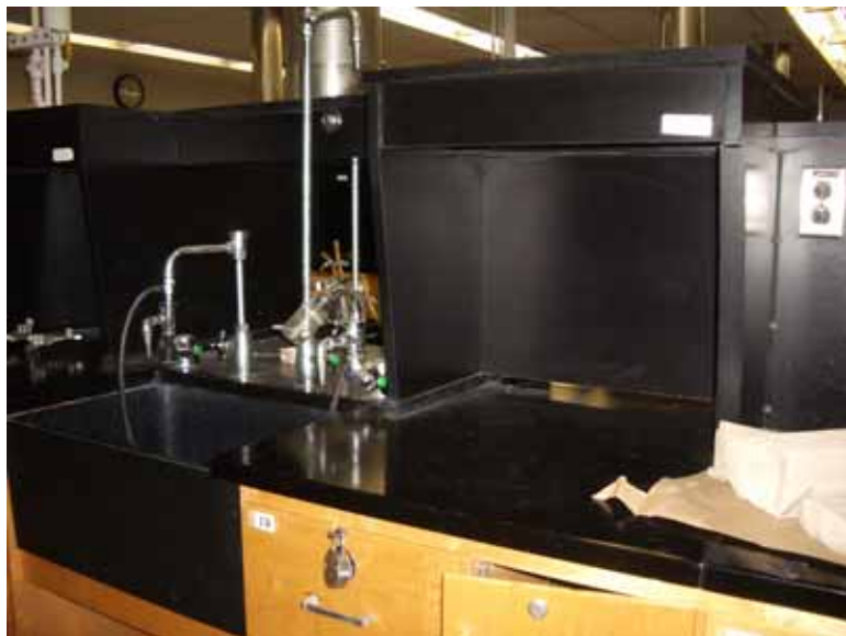
Figure 4: FUME COLLECTION BOXES OBSTRUCT INSTRUCTORS' SIGHT-LINES
