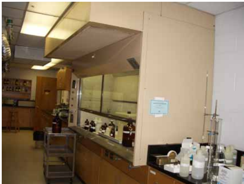
Figure 5: EXISTING CHEMICAL FUME HOOD – AUXILIARY AIR TYPE
