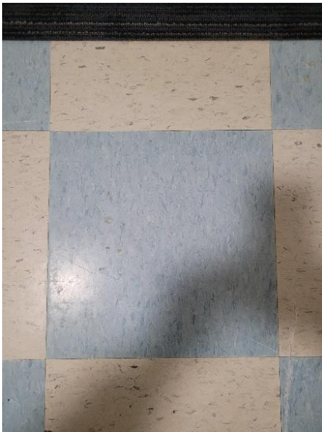
Photo #11 12"x12" Blue Floor Tile and Asbestos-Containing Mastic (Under Carpet) (HA 30)
