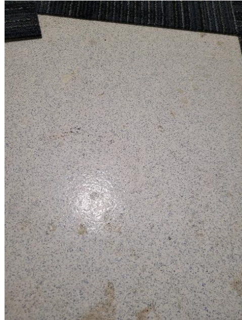
Photo #10 White with Blue Speckles Sheet Flooring and Asbestos-Containing Mastic (Under Carpet) (HA 29)
