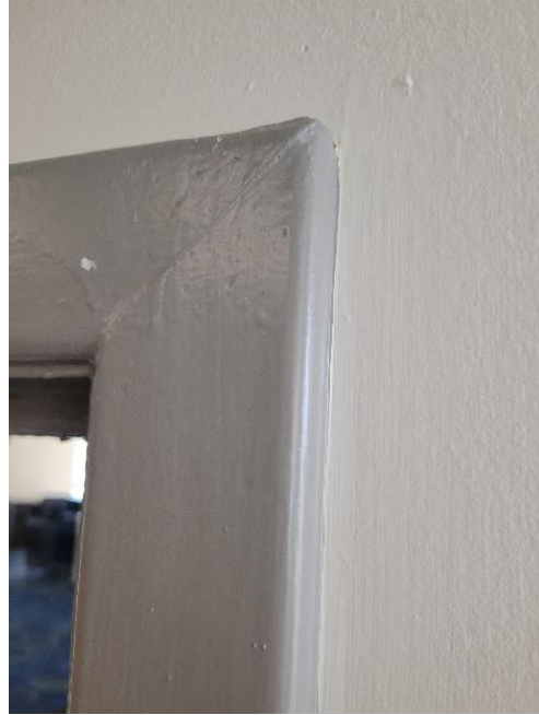
Photo #22 Asbestos-Containing Interior Door Caulk (Ground Floor) (HA 65)
