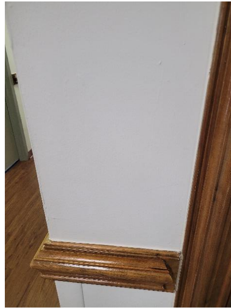
Photo #6 <1% Asbestos (Composite) Drywall and Joint Compound (1 st Floor) (HA 11)
