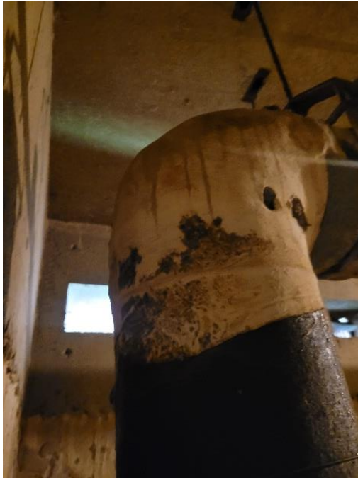
Photo #25 Asbestos-Containing 8" Pipe Hard Mudded Elbow (HA 75)
